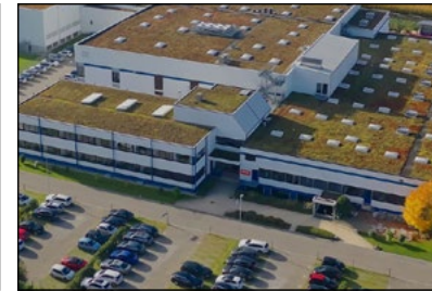
IQAir AG Technology Center Steinach, Switzerland
